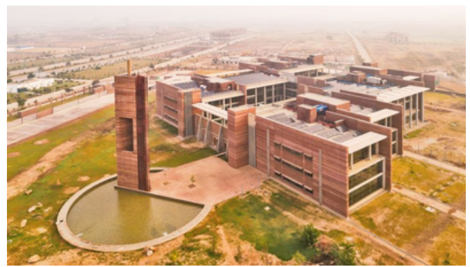
Image 9. Telenor Headquarters, Islamabad (The tallest building using rammed earth materials) (Source: Sirewall)
